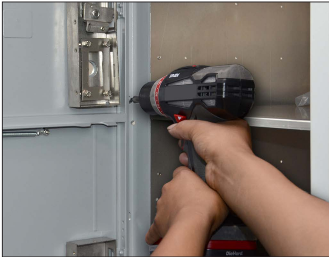
Figure 4F – 4C Connector Bar is now attached to parcel locker unit
