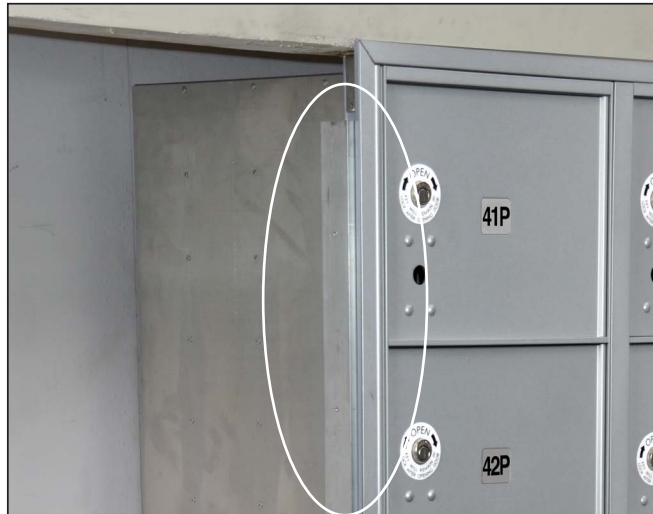
Figure 4F – 4C Connector Bar is now attached to parcel locker unit
